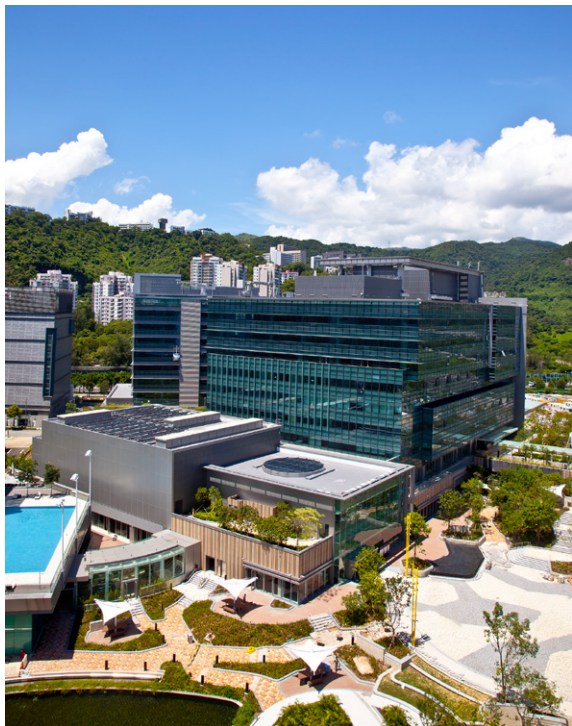
Science Park Phase 3 a&b Building 12W
