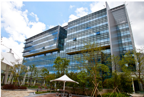
Science Park Phase 3 a&b Building 16W
